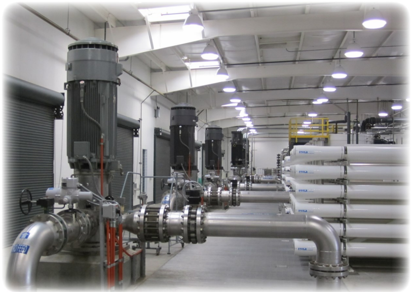
Chino II Desalter Facility
